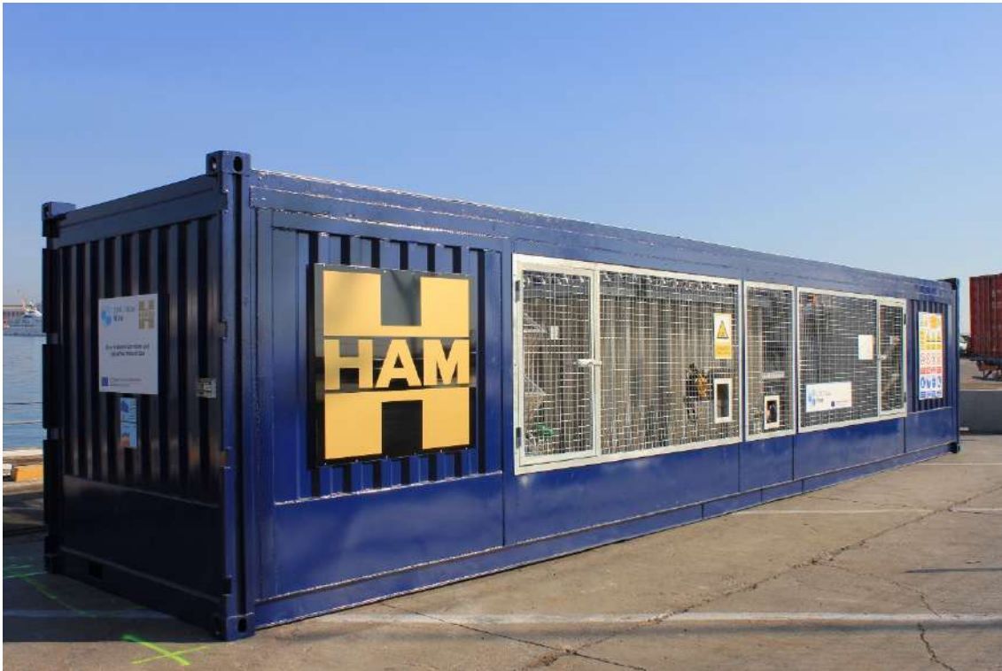
Figure 2. Module container of the LNG tanks and regasification plant (HAM).
