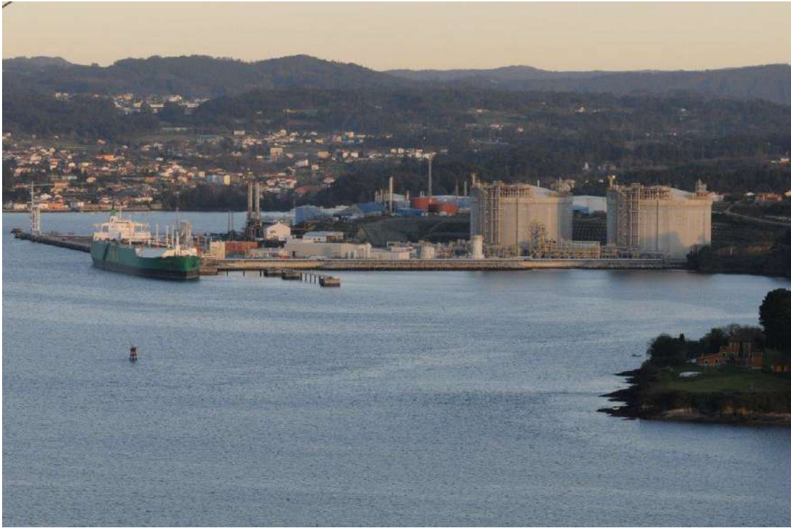
Figure 25. View of the plant of Reganosa
